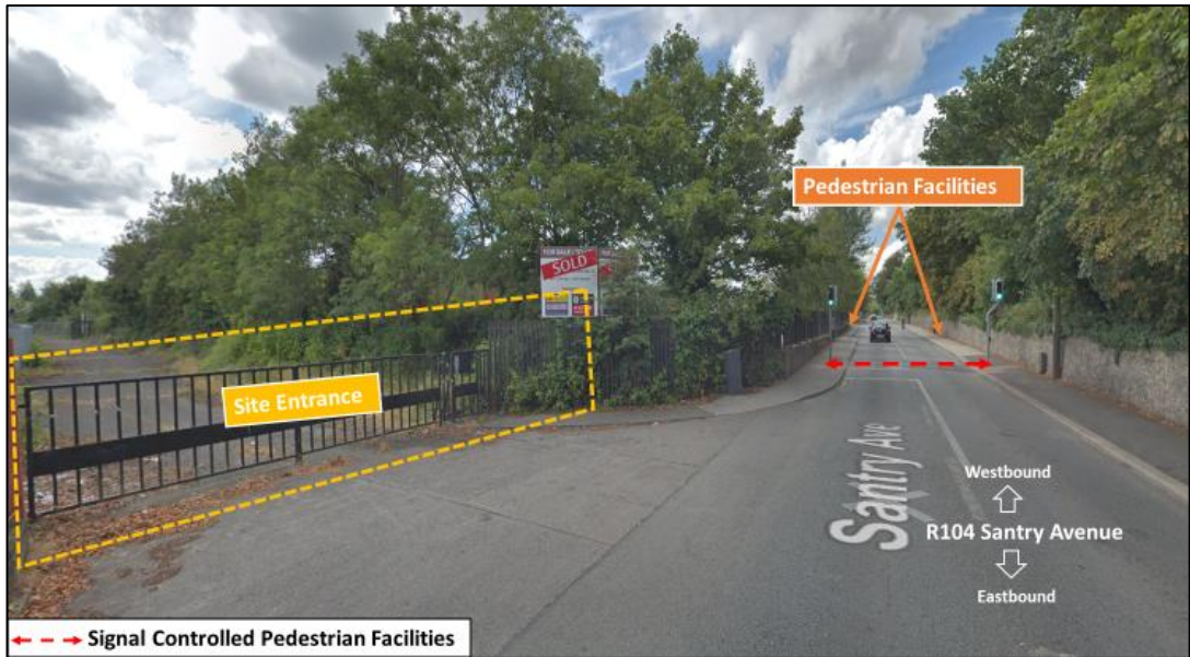
Figure 2.6: Pedestrian Facilities at Santry Avenue
